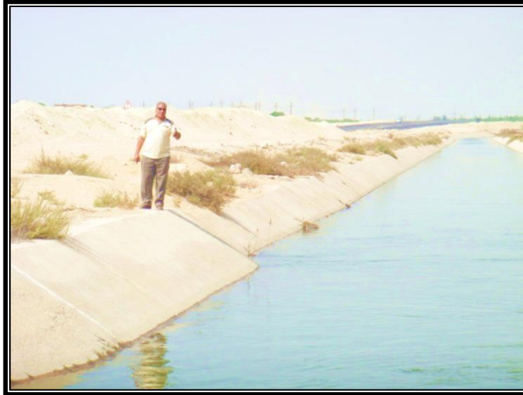
Picture 5: Sand Drift along Sheikh Zayed Canal, East of the SCLR
