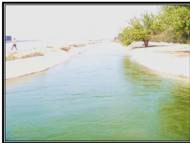
Picture 3: Sheikh Zayed Canal, East of the SCLR
