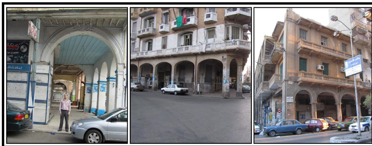
Figure 12. Constructing Arcades with Arched Vaults (Al-Bauki) in Old Residential Buildings in Port Said
