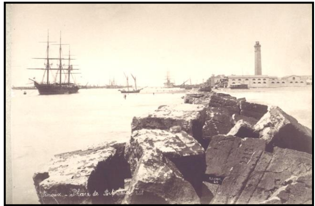
Figure 4. The Artificial Rocks, Used to Erect Two Breakwaters, Was Made in the Form of Blocks
