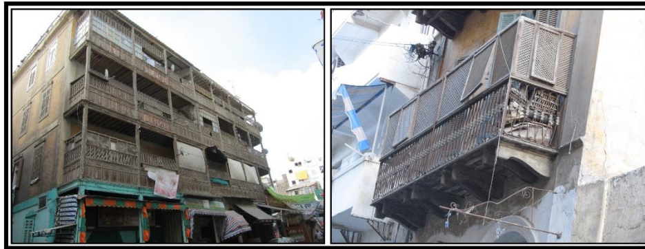
Figure 16. Balconies and Mashrabiyas in the Old Residential Buildings in Port Said
