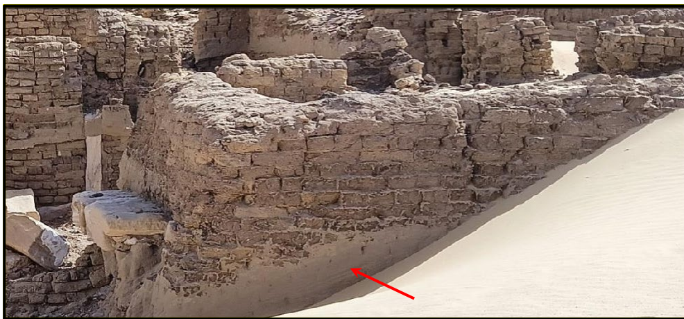
Figure 8. The Protective Effects of Sand Burial on the Doush Temple Structure. “Note that the buried sections still retain their outer plaster layer.”
