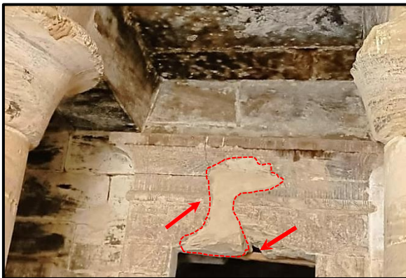
Figure 19. Improper Restoration Techniques Applied to Weathered Sandstone of the Doush Temple
