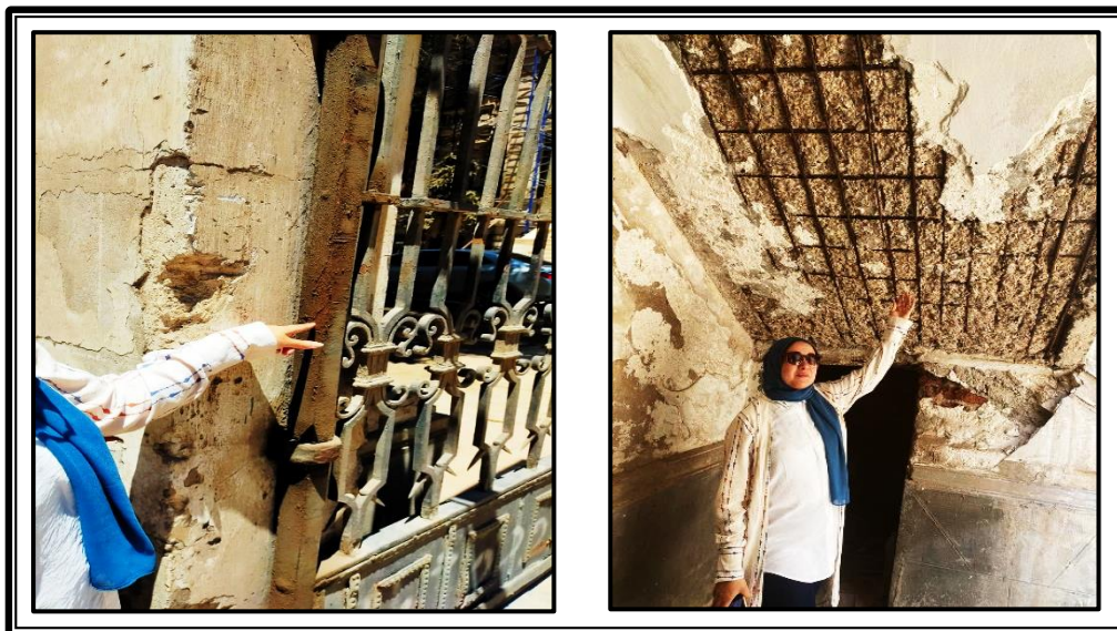
Figure 24. Rusting iron in the Al-Shinawi Palace building in Mansoura City
