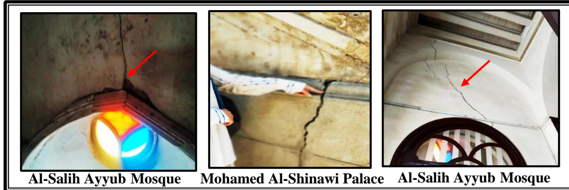
Figure 23. Cracks in some heritage buildings of Mansoura City
